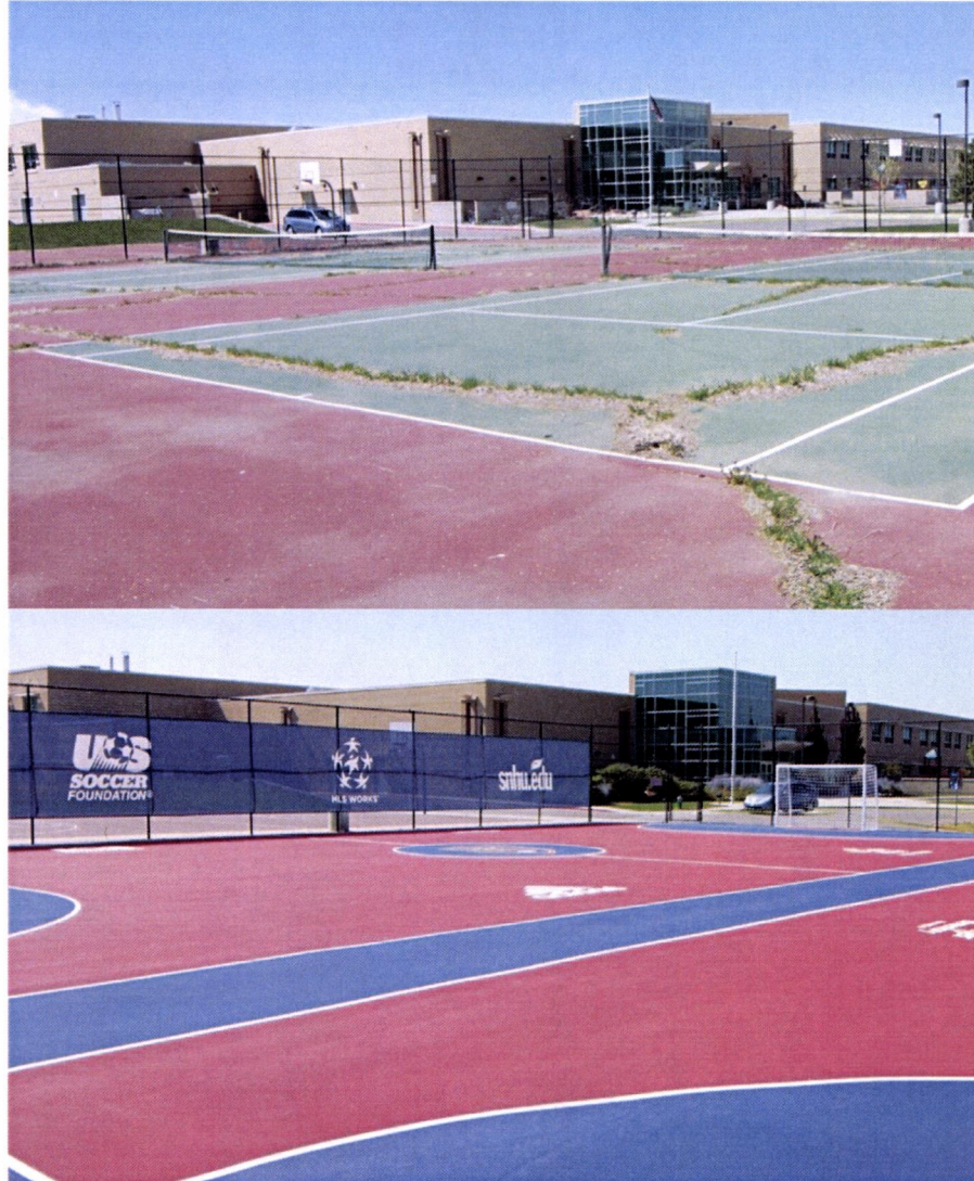
Granger Elementary School
