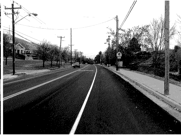
Fig.3- Southbound view from proposed access
