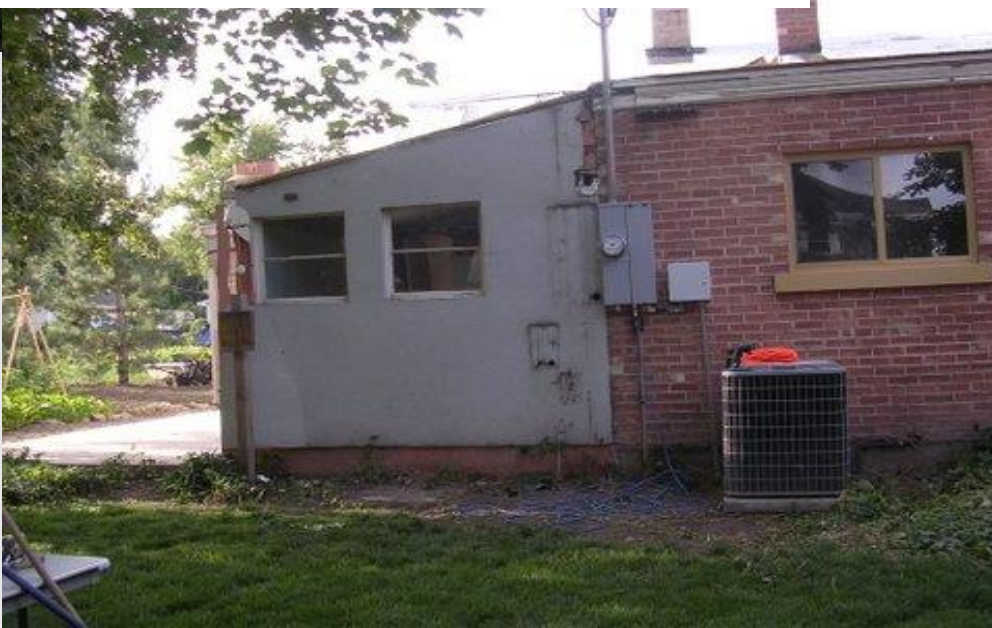
1960's addition being removed - east side
