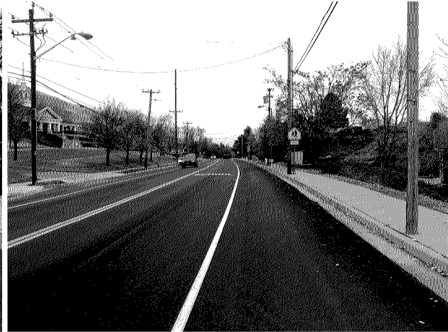
Fig.3- Southbound view from proposed access
