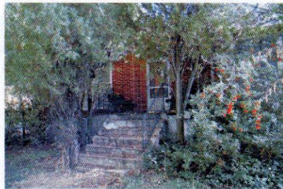
221 South Main Street Contributing Property
