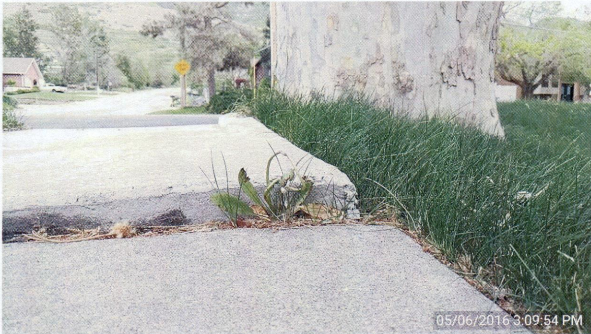
Figure 1 1-3" Fault
