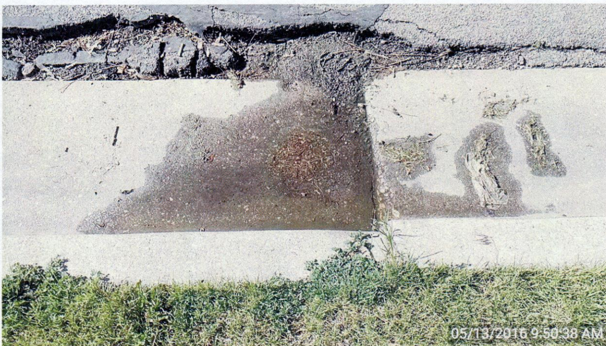
Figure 6 Curb Misalignment
