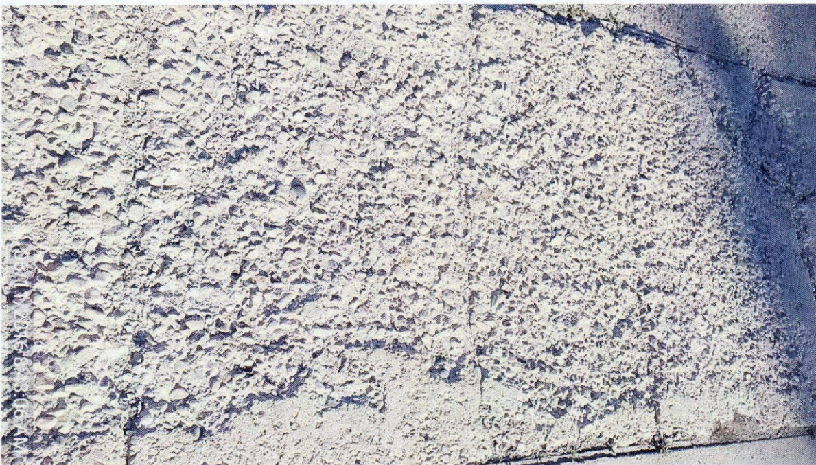
Figure 4 Spalling
