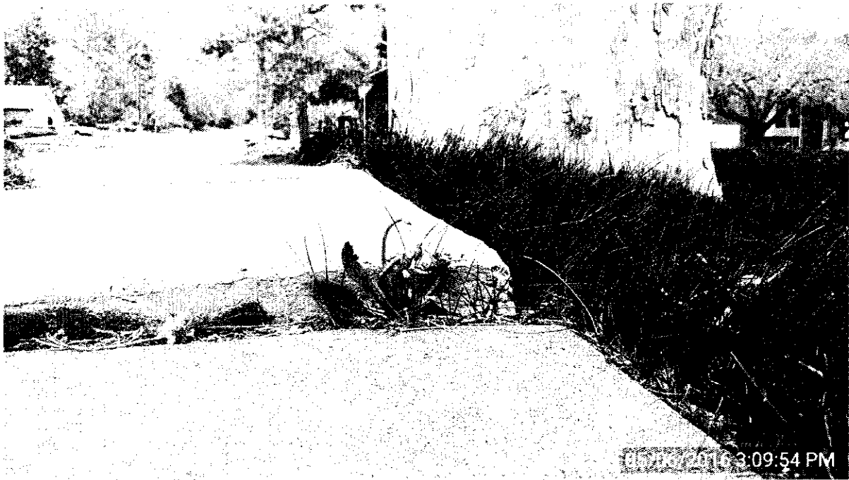
Figure 1 1-3" Fault
