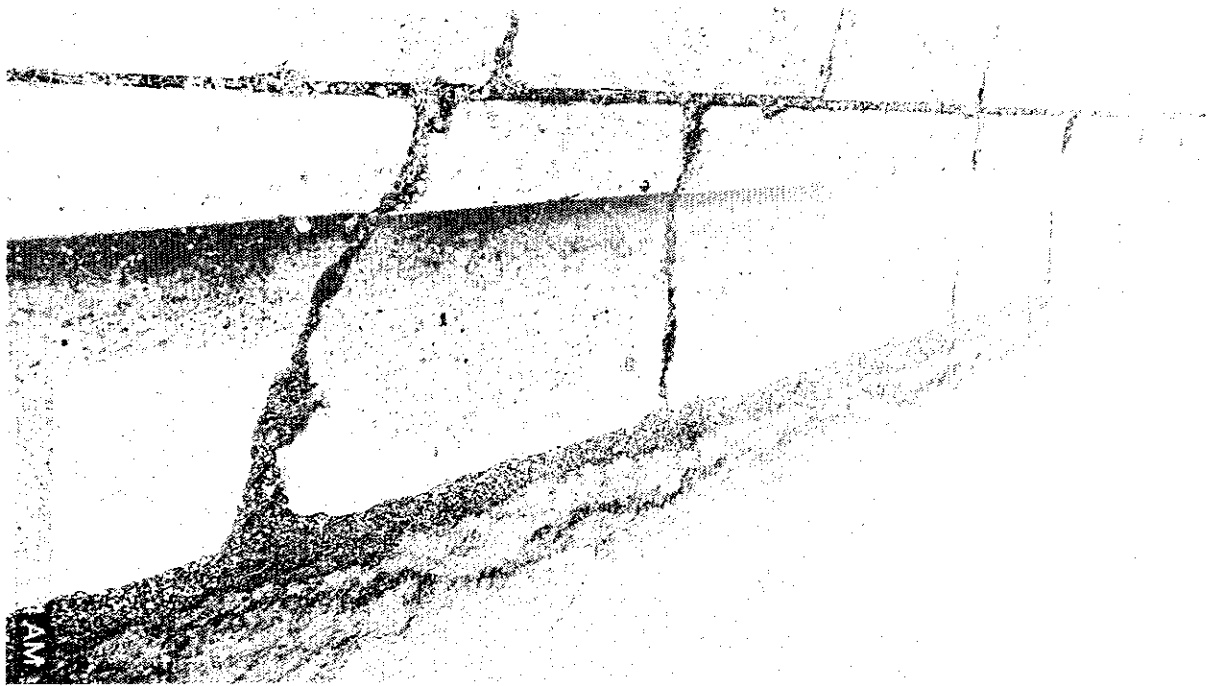
Figure 7 Curb Break Down
