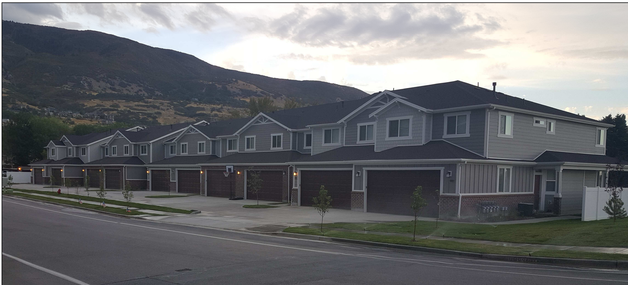
Kestrel Bay Townhomes 155 West 620 South, Farmington, Utah Designed and Constructed by Scott and Angie Balling
