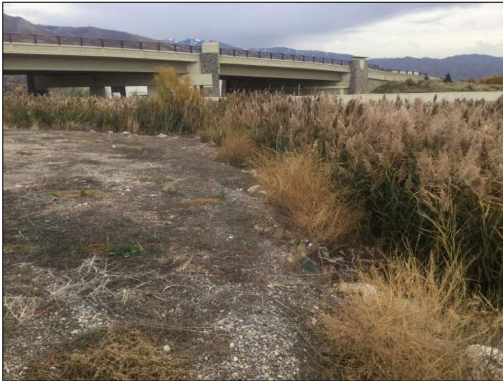
Photo 1. View southeast of the boundary between the wetland and the gravel lot.
