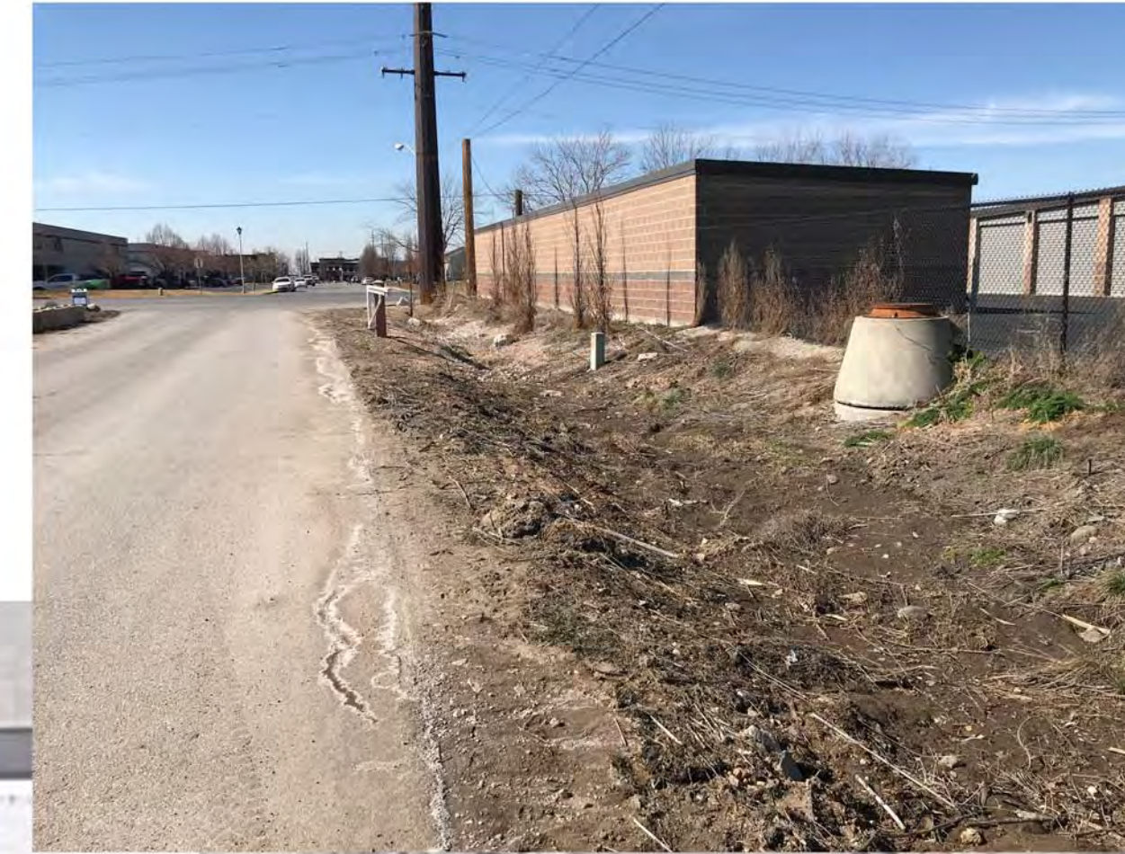
EXISITNG DITCH AT W 75 N
