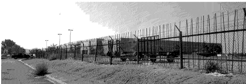
Figure 2 Existing fence on east side of property (photo facing south)
